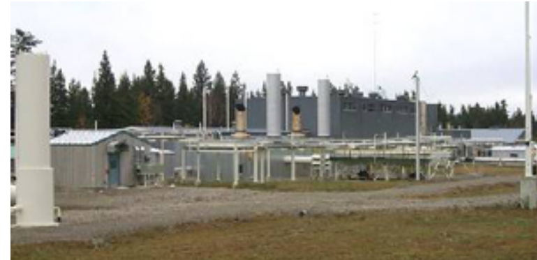
Pumping station for a natural gas pipeline Source: Duke Energy Gas Transmission Canada
