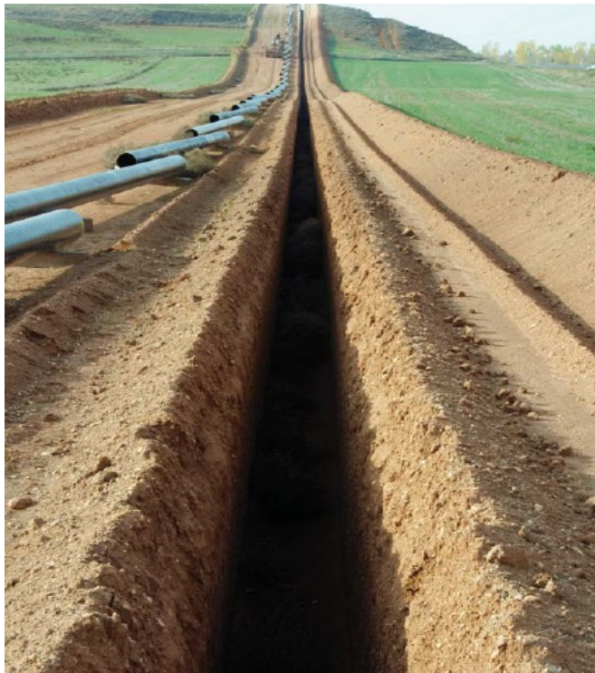
Natural Gas Transmission Pipeline and Pumping Station
